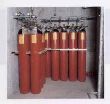
ensure that the correct amount of Argonite is released effectively. Argonite's inerting and extinguishing properties act quickly to eliminate the fire.
